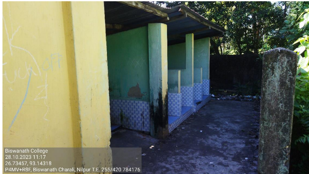
Boys' Toilet in Arts & Science Block
